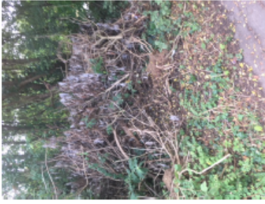
PHOTO SHOWS POSITION C ON EXISTING EXAMPLE OF LACK OF MAINTENANCE
